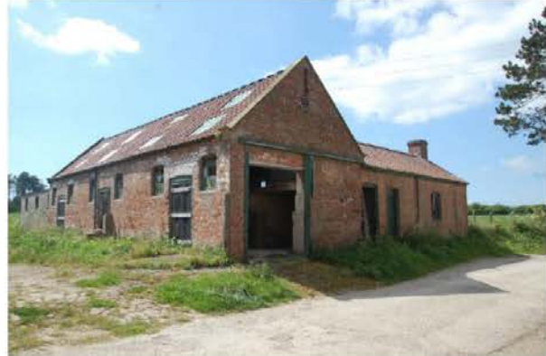
Stables from north east
