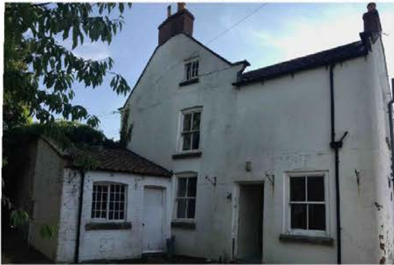
East side of Home farm house (plot 1)
