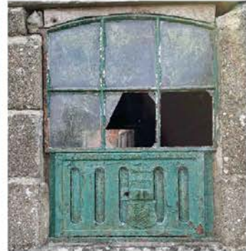
Iron window vents
